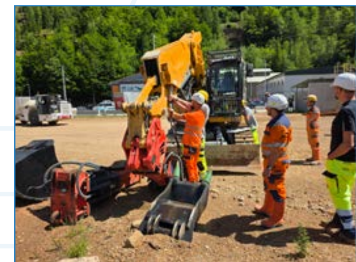
Tunnel-construction-technician-training at ZaB/Eisernerz on the yellow Fox
