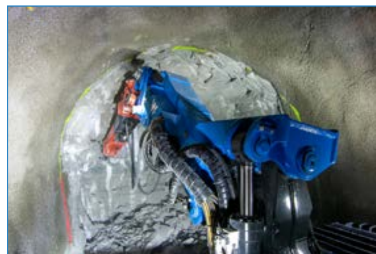
TU-breaker in action with the mini Badger
