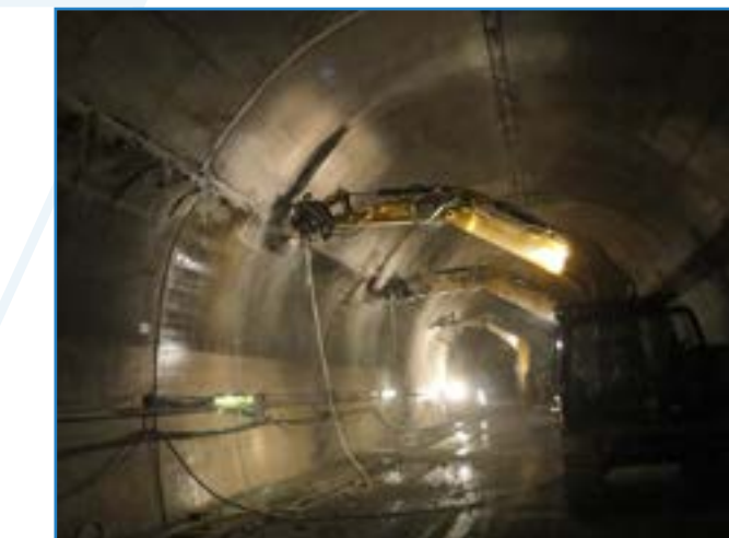
Hydraulic cutter in tunneling
