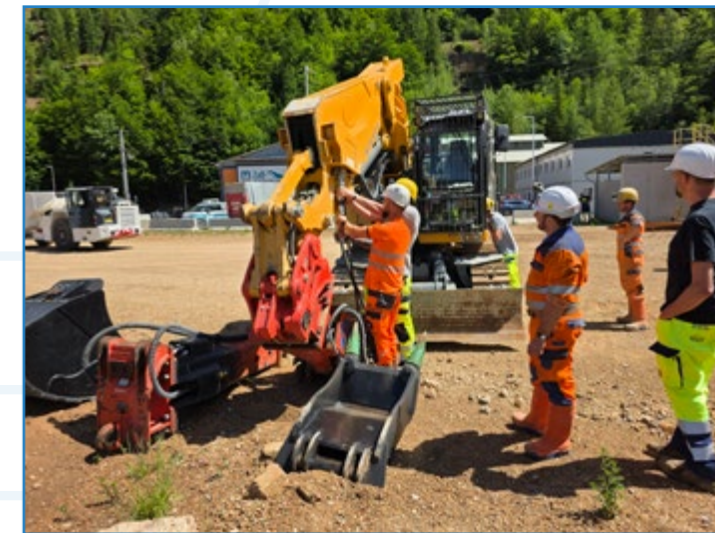
Tunnel-construction-technician-training at ZaB/Eisenerz on the yellow Fox
