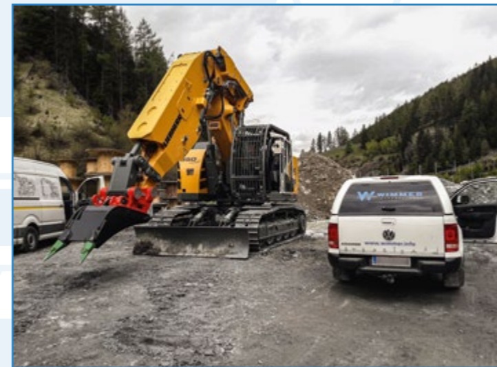
Quick coupler installation on site by our fitters and service technicians
