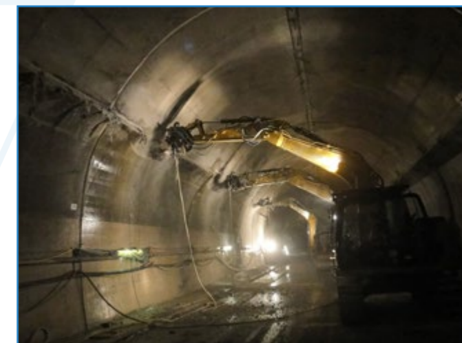
Hydraulic cutter in tunneling
