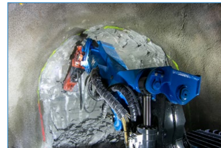
TU-breaker in action with the mini Badger
